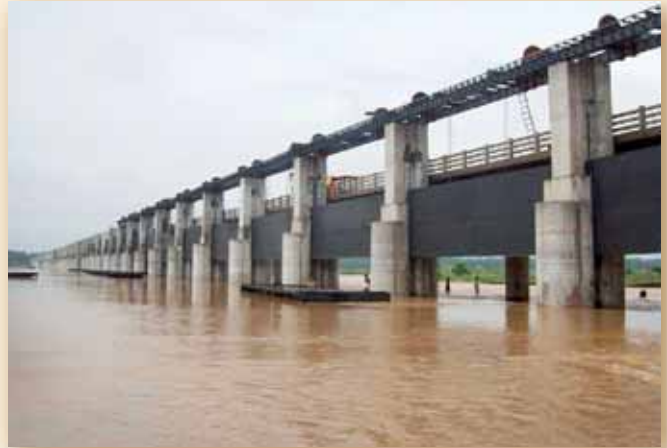
Regulator Cum Bridge, Chamravattam, Kerala
